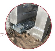
Here's an example of carriages mounted on post brackets instead of a pad:
