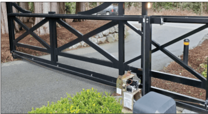
Best: “X” bracing in each section of the gate, which is best for large, heavy gates.
