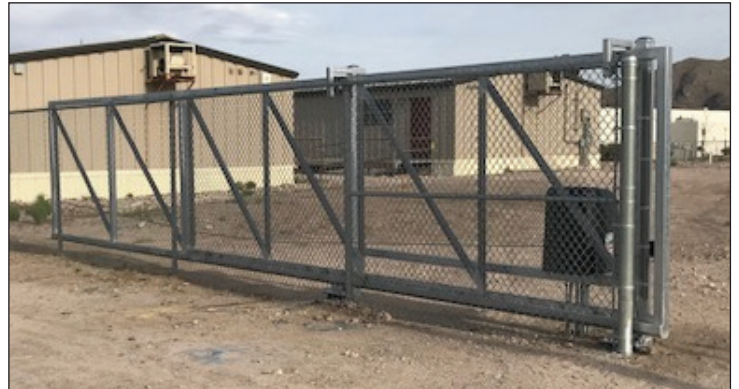
Better: One diagonal brace in each gate section, is recommended for large gates with a 30 ft or greater opening.
