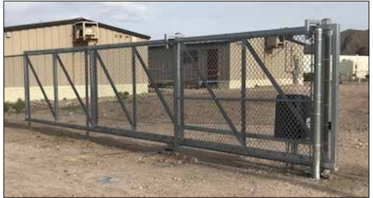
Diagonal bracing in each section should be used for large gates with a 30 ft or greater opening.
