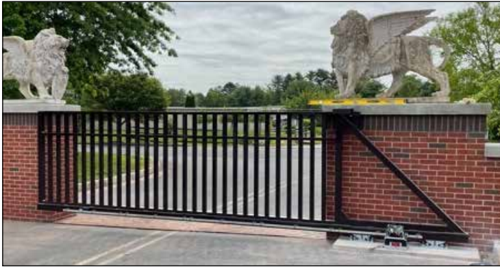
Diagonal trussing in the vertical dimension is needed for all gates. A simple diagonal in the tail section will work for many "smaller" gates.
