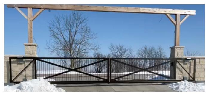
This large entrance required sturdy gates with minimal visible hardware. This client decided to use DuraGates Aluminum Track Model, CGA-350.5P. The gate cantilevers over the driveway instead of having V-Groove track mounted on the ground in the entrance. When the gates are both open, they tuck nicely behind the two brick walls. By choosing the aluminum model, there is no chance of rust or corrosion, making these gates a low maintenance addition to the property.
