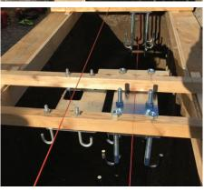
**Note:** The top of the bolt/tie rod should stick out of the cement at least 2". Keep nut on top of concrete, do not sink in.
