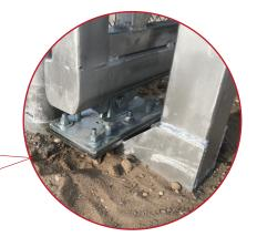
Here's an example of carriages mounted on post brackets instead of a pad:
