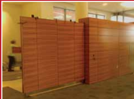
Moving wall to separate the Pediatric lobby at Golisano Children's Hospital in Rochester, NY.
